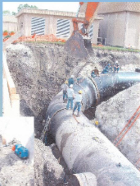
Richland Chambers Expansion Ennis, TX Archer - Western 120 of 54" - 120" Butt Straps
