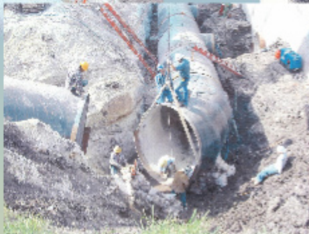
Richland Chambers Expansion Ennis, TX Archer - Western 120 of 54" - 120" Butt Straps
