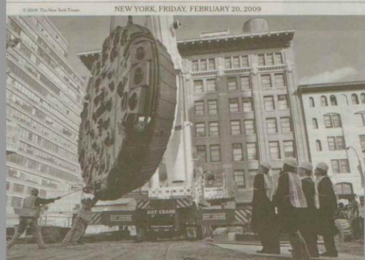
Digging to Times Square, an Inch at a Time New York City and transit officials attended a ceremony Thursday at 25th Street and 11th Avenue, where a 22-foot cutter head was lowered into the ground. The cutter will be mounted on a 100-ton boring machine, which will extend the subway's No. 7 line.
