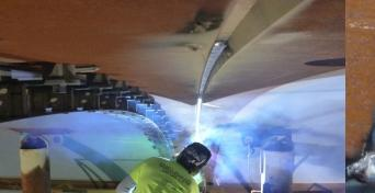
Automatic and Semi-Automatic FCAW Welding
