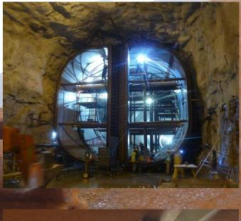
Over 937 m (3076 ft) of CJP tunnel welds performed
