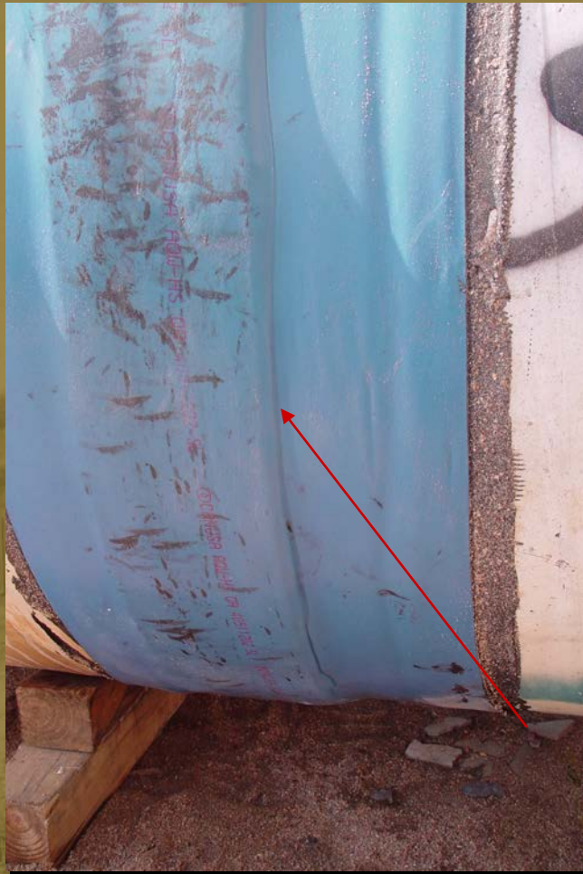
Step down edge recovery due to heat effect at bell and spigot interface
